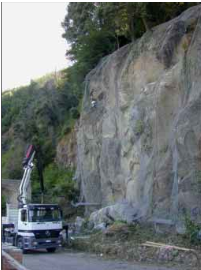
Securing basalt cliff by Nemi town gate in July 2001
