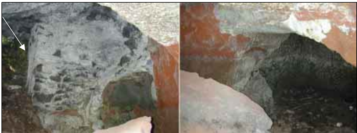
The westernmost cave. Left: West side close to entrance with masonry structure. Arrow indicates the location of the former door to the chapel. Right: Interior of the westernmost cave. Red colour is probably algae.
