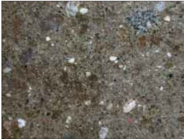
Peperino stone on the floor of the chapel with its characteristic speckled appearance (width of field c. 10 cm)
